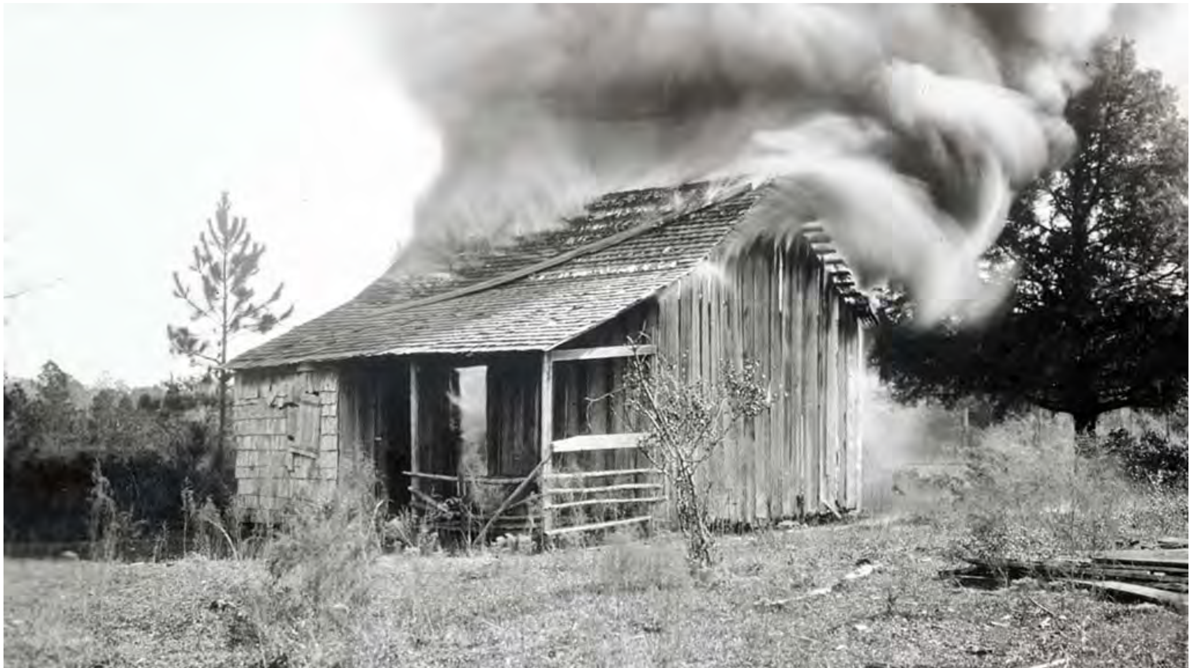
Rosewood Cabin Burning
