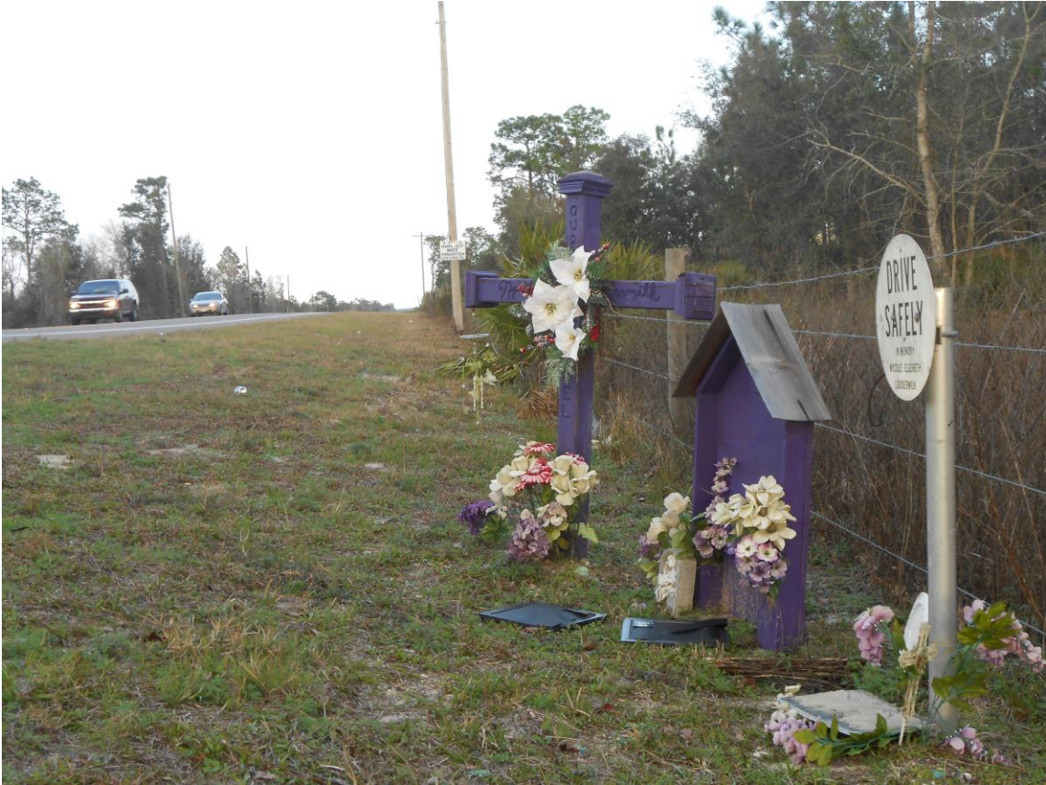
Hwy 24, shown above, is on a raised piece of land. This photo shows the size of the roadside shoulders before the lands becomes swamp.
